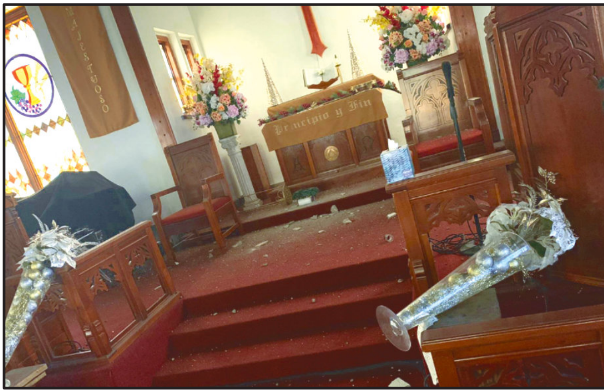
The Methodist Church of the Resurrection in Ponce, Puerto Rico, suffered extensive damage in a series of earthquakes that have rattled the area since Dec. 28. Photo courtesy of the Methodist Church of Puerto Rico.
